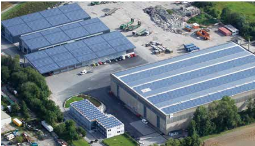
Novatech | Michelfeld-Erlin - Germany System: 1,4 MW | Solar fastener System
